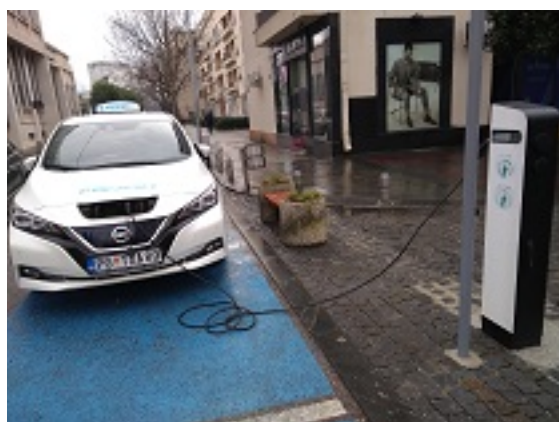
Podgorica – city center EV charging station (2 ports, 22 kW and 11 kW) with new EV taxi charging. Charging station supported by TCNTM .
